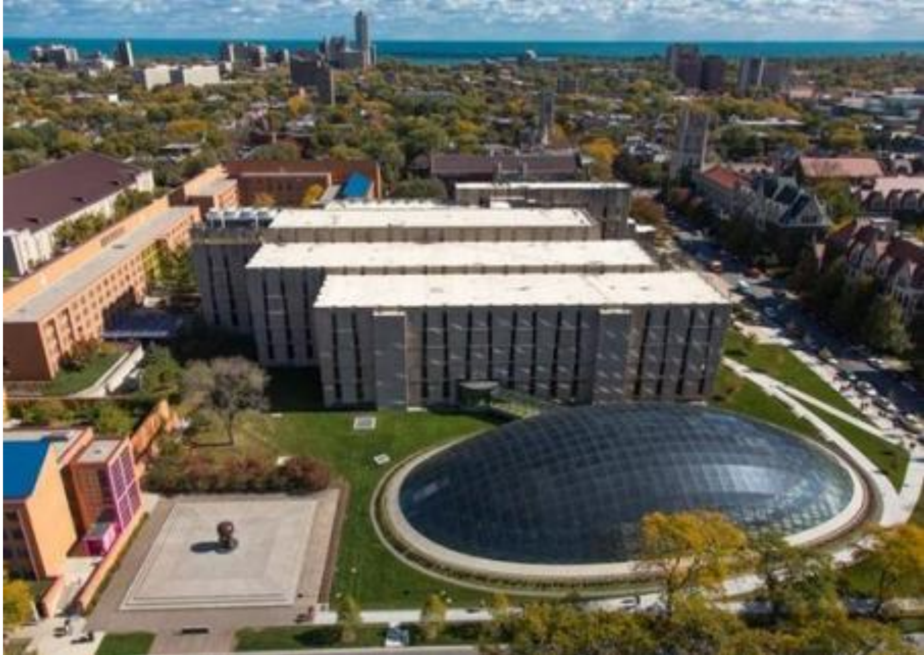
EXAMPLE OF UNDERGROUND BUILDING – REGENSTEIN LIBRARY AT THE UNIVERSITY OF CHICAGO
